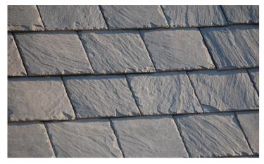
Domiz slate is guarried from the Rozadais geological formation within the province of Orense in north-west Spain. The geological composition of the Domiz slate demonstrates a range of properties that make it suitable for high-performance roofing slates.
