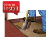
Dig trench 100mm wide by 210mm deep for channel. Remove cap from outlet.
