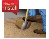
Dig trench, allowing for width of channel plus 100mm each side for concrete haunch. Trench depth should allow for channel depth plus 100mm for concrete bedding. Also allow for 100mm concrete around and beneath sump unit. Mark finishing height with fixed line 3mm below final surface. Lav 100mm (min) bed of concrete.
