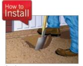
Dig trench 318mm wide (218mm wide if against a structure) by 200mm deep for channel (400mm deep for sump). Mark finishing height with fixed line 3mm below final surface. Lay 100mm (min.) bed of concrete.
