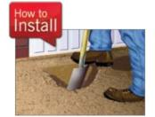
Dig trench 325mm wide (225mm wide if against a structure) by 208mm deep for channel (408mm deep for sump). Mark finishing height with fixed line 3mm below final surface. Lay 50mm (min.) bed of concrete.
