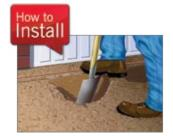
Dig trench 318mm wide (218mm wide if against a structure) by 200mm deep for channel (400mm deep for sump). Mark finishing height with fixed line 3mm below final surface. Lay 100mm (min.) bed of
