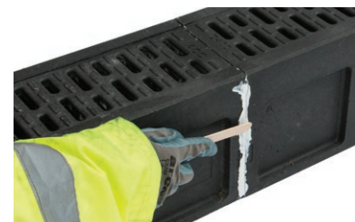
Pipe connection to endcap
