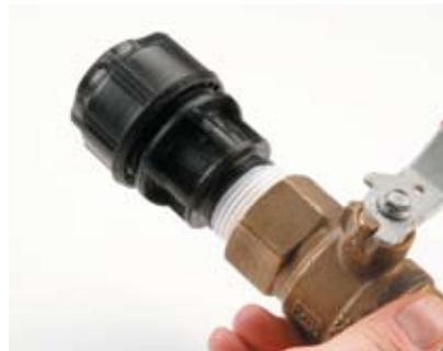
2. Using your hands, screw the thread of the Male Adapter into the valve until firm.
