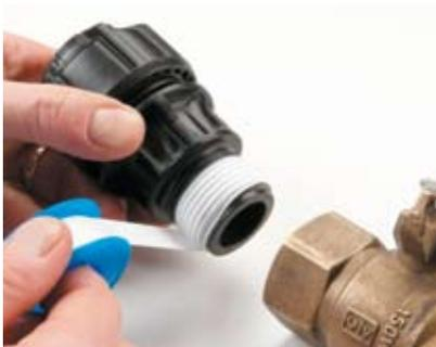
1. Apply PTFE tape or suitable\* sealant to the plastic thread ensuring sufficient is applied to ensure a watertight seal.
