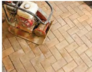
An appropriate plate compactor is used to compact the paving blocks fully. Any joints not full after compaction is complete are topped up by sweeping more sand into them.
