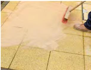
The jointing material (Kilsaran Jointing Sand) is carefully swept into the joints.
