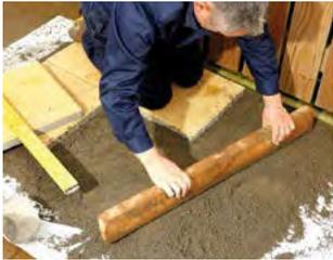
A sand/cement bedding mix is used as the laying course and this is screeded off to the correct levels. We recommend the use of our pre-mixed Patio Bedding Mix (in 25kg bags) for domestic patio areas.
