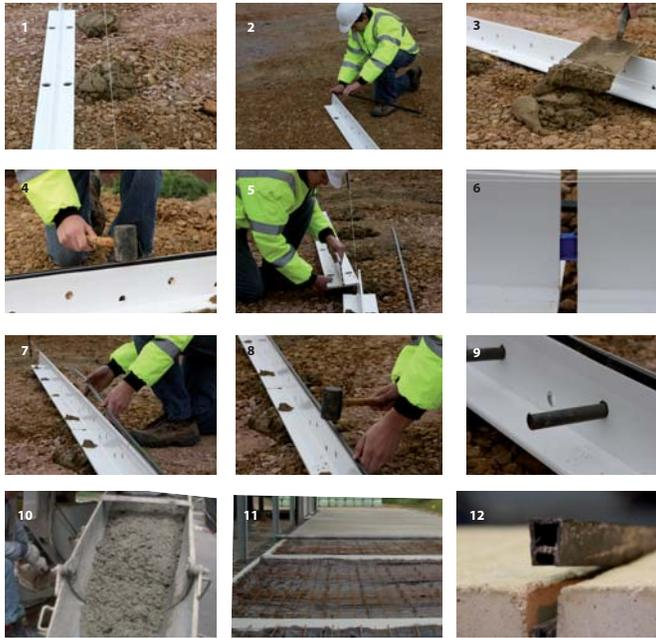
K-FORM is ideal for concrete slabs of various thicknesses. The rail is simply laid on a lean mix or mortar bed to the required finished height.
