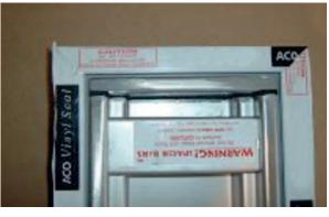
Picture shows the rigid extrusion cut and fitted prior to the fitting of the black flexible seal.
