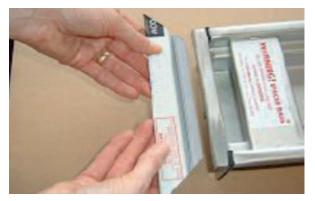
Cut grey rigid seal extrusion to suit ensuring any mitres are cut accurately otherwise pressure points may appear in the finished fioor in use.
