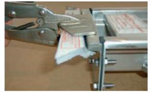
Using Sheet Plier Grip Wrench clip the rigid seal extrusion into the underside of channel.
