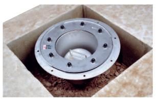
Position gully and check levels. Keep loose materials clear of gully.
