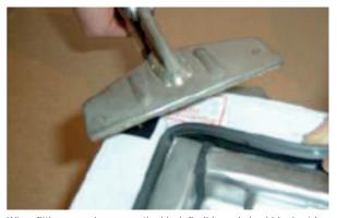
When fitting around a corner, the black flexible seal should be kept in one piece to minimise joints.
