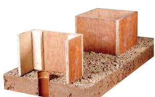
Construct shutters, position and mark concrete level. Leaving the shutters long allows easy removal after concrete pour.
