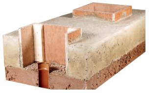
Pour concrete slab and leave for 24 hours before removing shutters.
