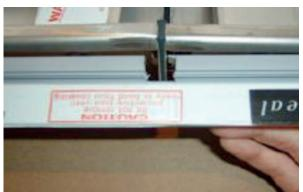
Where there are joint plates in the channel run cut a notch out of the rigid seal extrusion as shown to enable the extrusion to be clipped to the underside of the channel.
