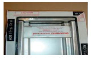
Picture shows the rigid seal extrusion and black flexible seal fitted prior to screeding / back filling.
