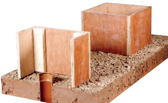
Construct shutters, position and mark concrete level. Leaving the shutters long allows easy removal after concrete pour.
