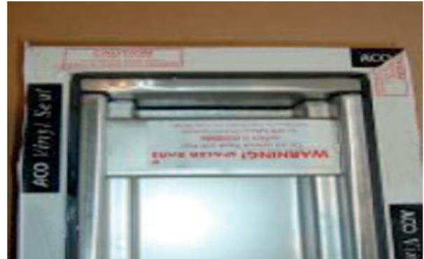
Picture shows the rigid seal extrusion and black flexible seal fitted prior to screeding / back filling.
