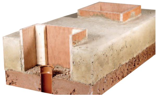
Pour concrete slab and leave for 24 hours before removing shutters.
