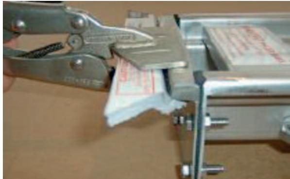
Using Sheet Plier Grip Wrench clip the rigid seal extrusion into the underside of channel.
