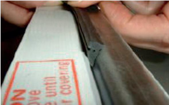
Insert the black flexible seal inbetween channel edge and rigid seal extrusion making sure that the curved concave section of the seal faces TOWARDS the channel edge and that the groove in the black flexible seal engages with the notch on the rigid seal extrusion. (It may help to lubricate the flexible seal when inserting using a water soluble soapy solution).
