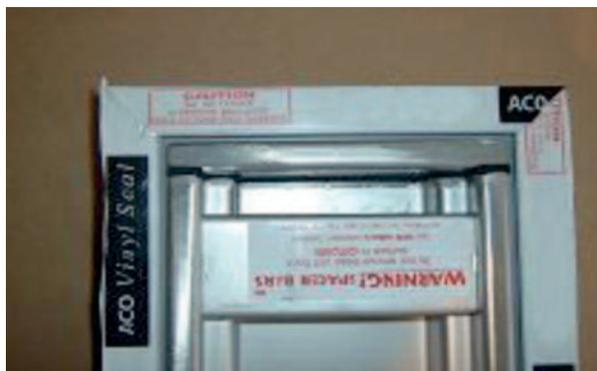
Picture shows the rigid extrusion cut and fitted prior to the fitting of the black flexible seal.
