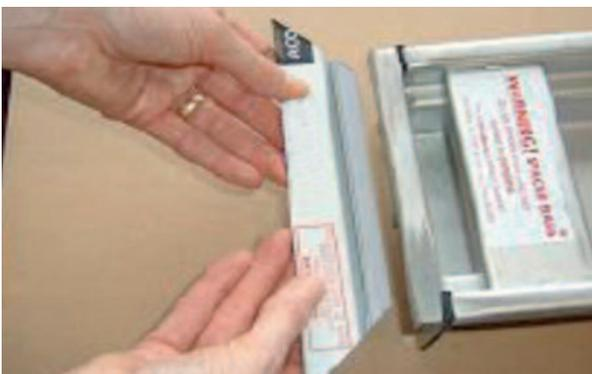
Cut grey rigid seal extrusion to suit ensuring any mitres are cut accurately otherwise pressure points may appear in the finished floor in use.
