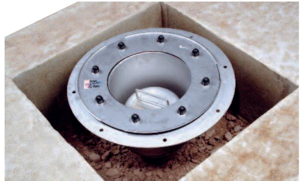
Position gully and check levels. Keep loose materials clear of gully.
