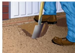
Dig trench 318mm wide (218mm wide if against a structure) by 278 mm deep for channel (483mm deep if installing sump unit). Mark finishing height with fixed line 3mm below final surface. Lay 100mm (min.) bed of C25 concrete.
