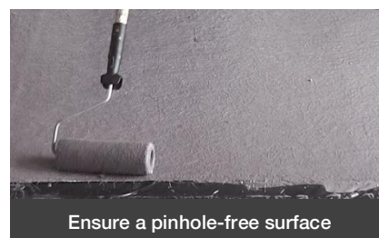
Wetting through the fibreglass CSM
